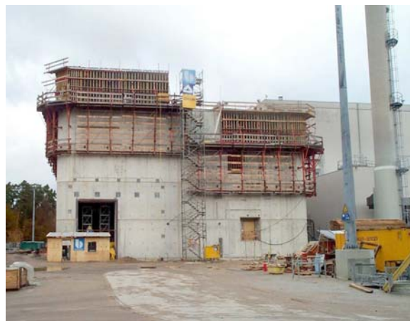
Fig. 2. Construction Site from South (Status November 2001)
