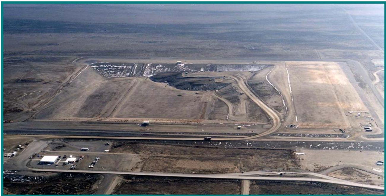
Fig. 3. The Bechtel Hanford-led ERC team operates the Environmental Restoration Disposal Facility.
