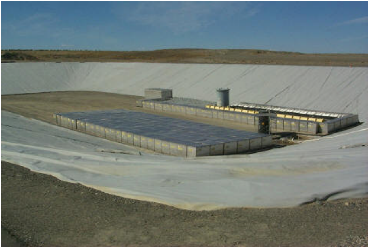
Fig. 1. Hanford MLLW Disposal Facility (Trench 34)
