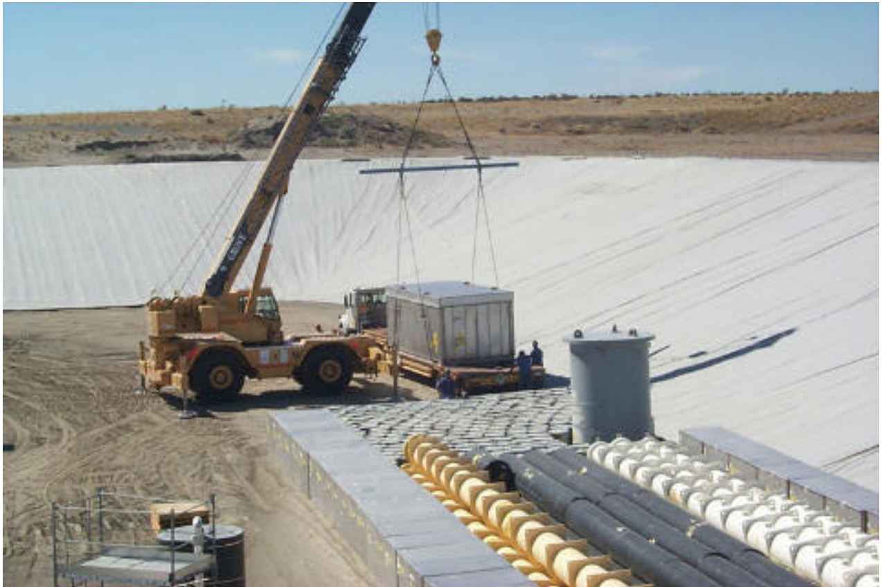
Fig. 2. Placement of Macroencapsulated Debris in Trench 34
