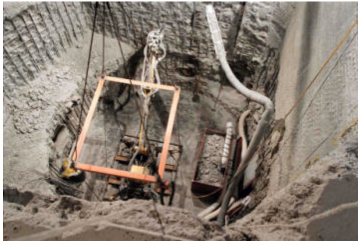
Fig. 3 - Concrete Removal in Reactor Cavity at YNPS
