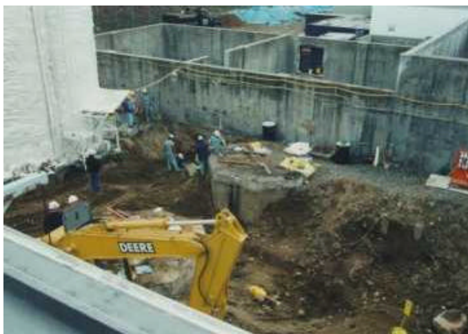
Fig. 2 - Soil Removal Near Waste Monitor Tanks at YNPS
