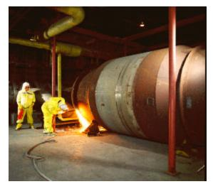
Fig. 2. Dismantling a Converter
