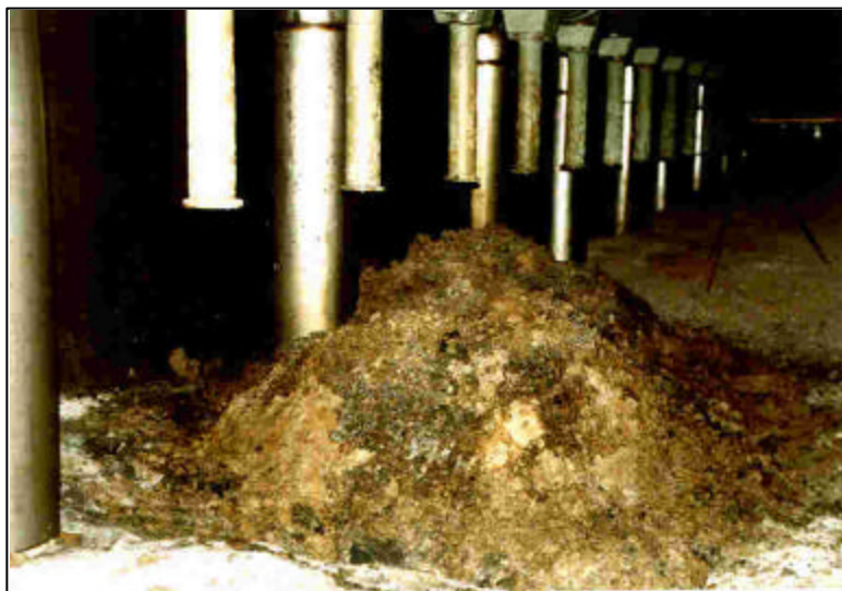
Fig. 2 Pile of Lava-Produced Fuel-Containing Material in Bubble Room Area
