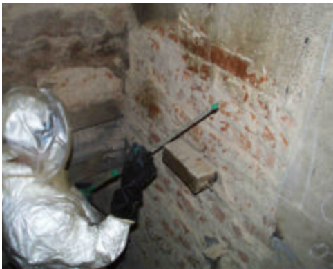
Fig 2. Application of dust-suppressing polymers
