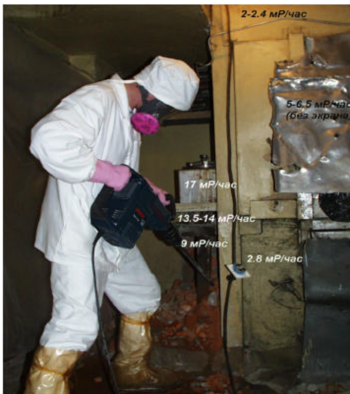
Fig. 4. Metering tank casing dismantling
