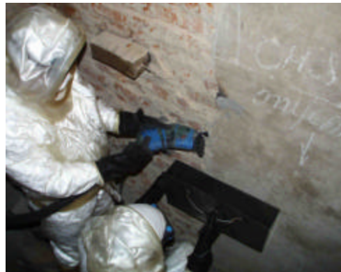
Fig 3. Demolishing of contaminated plaster.
