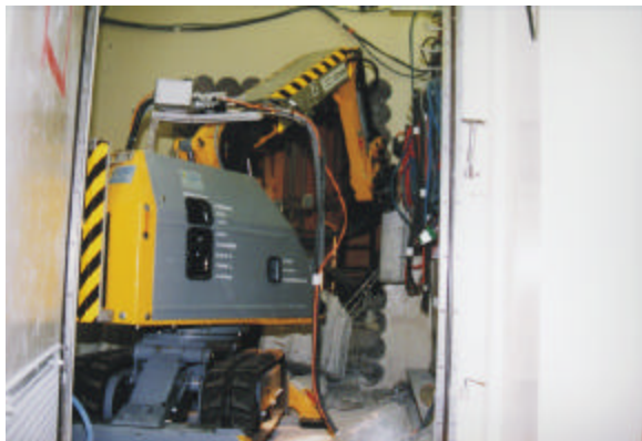
Fig. 1. Horizontal remote dismantling equipment (crawler digger Brokk 150) and control panel
