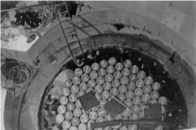
Fig. 2. View of RPV after dismantling of the rod-shaped components above the RPV
