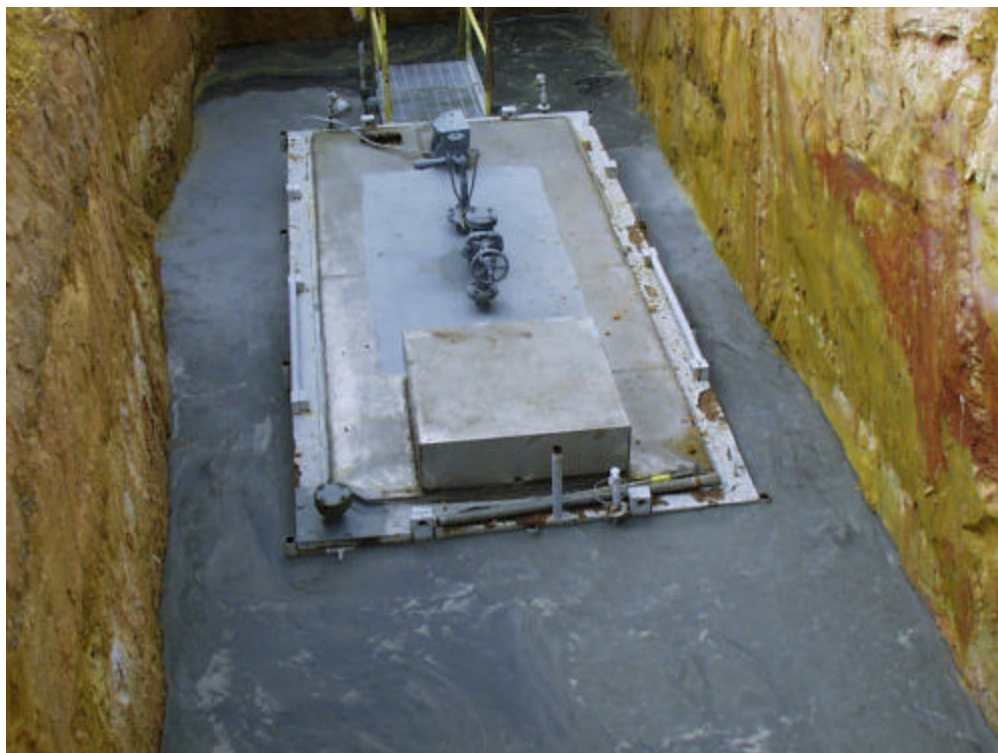
Fig. 3. Spent Solvent Trailer Partially Encased in Grout
