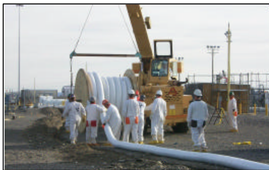
Fig. 1. Innovative double hose system rather than steel piping used to transfer single-shell tank liquids.
