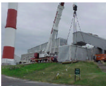
Fig. 2. Removal of above-ground ducts at the Brookhaven Graphite Research Reactor
