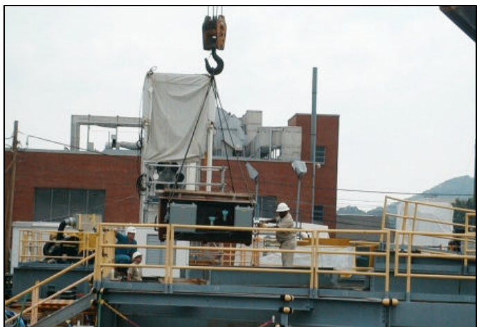
Fig. 14. Workers cut old tank mixer into small pieces for disposal.
