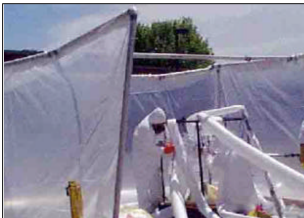
Fig. 18. Workers remove sludge from FFA Tanks.
