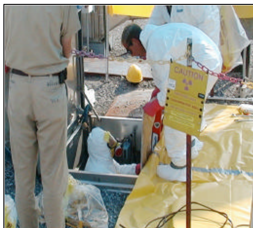
Fig. 13. Workers install waste retrieval and transfer equipment on another tank.
