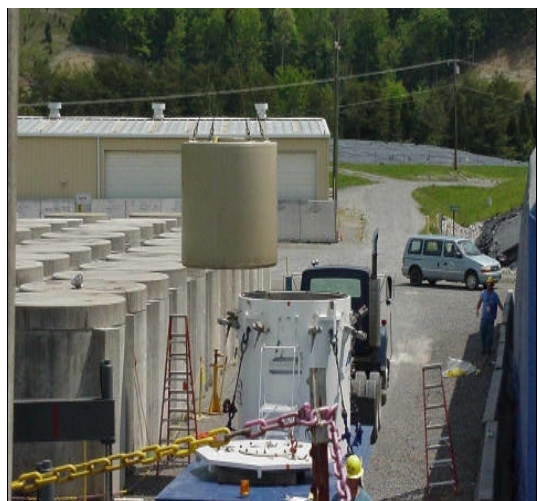
Fig. 20. The monolith is moved by crane to the shipping cask.
