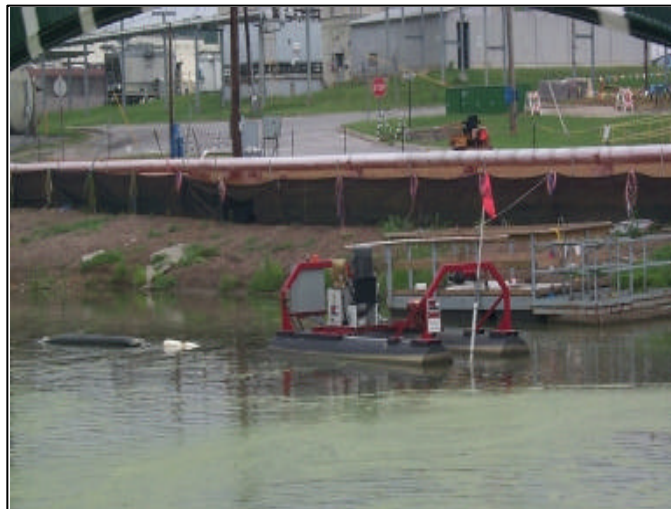
Fig. 17. Floating dredge removes sediments from surface impoundments.
