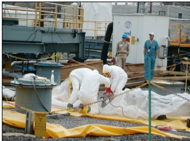
Fig. 15. Technician prepares to remove old waste piping from tank.
