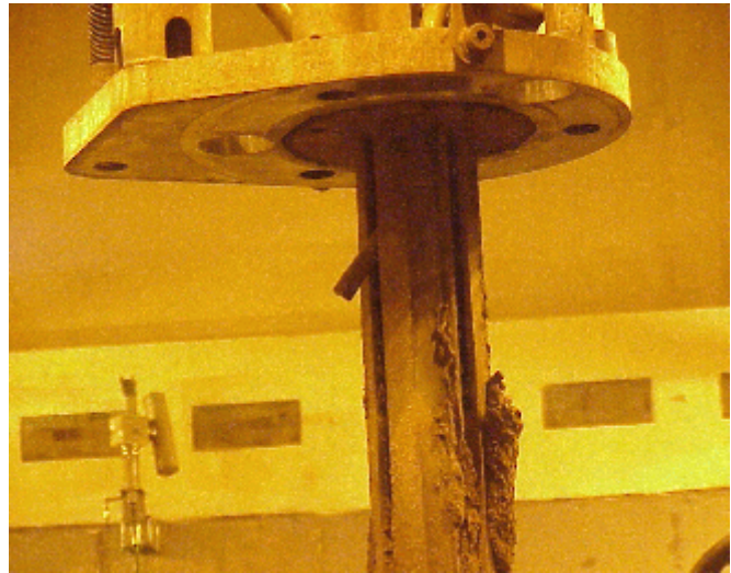
Fig. 5. Concentrator Air Displacement Slurry Pump with HLW Residue
