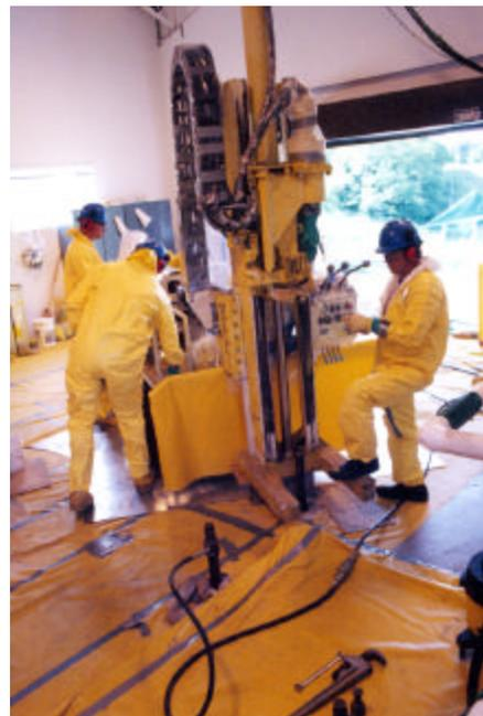
Fig. 2. CS injection at the BLIP
