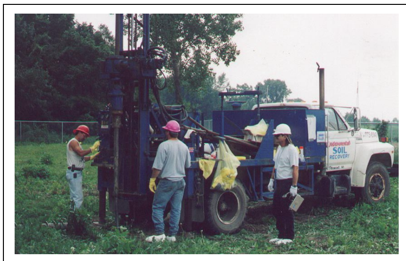
Figure 2. Conducting subsurface sampling at Breckenridge
