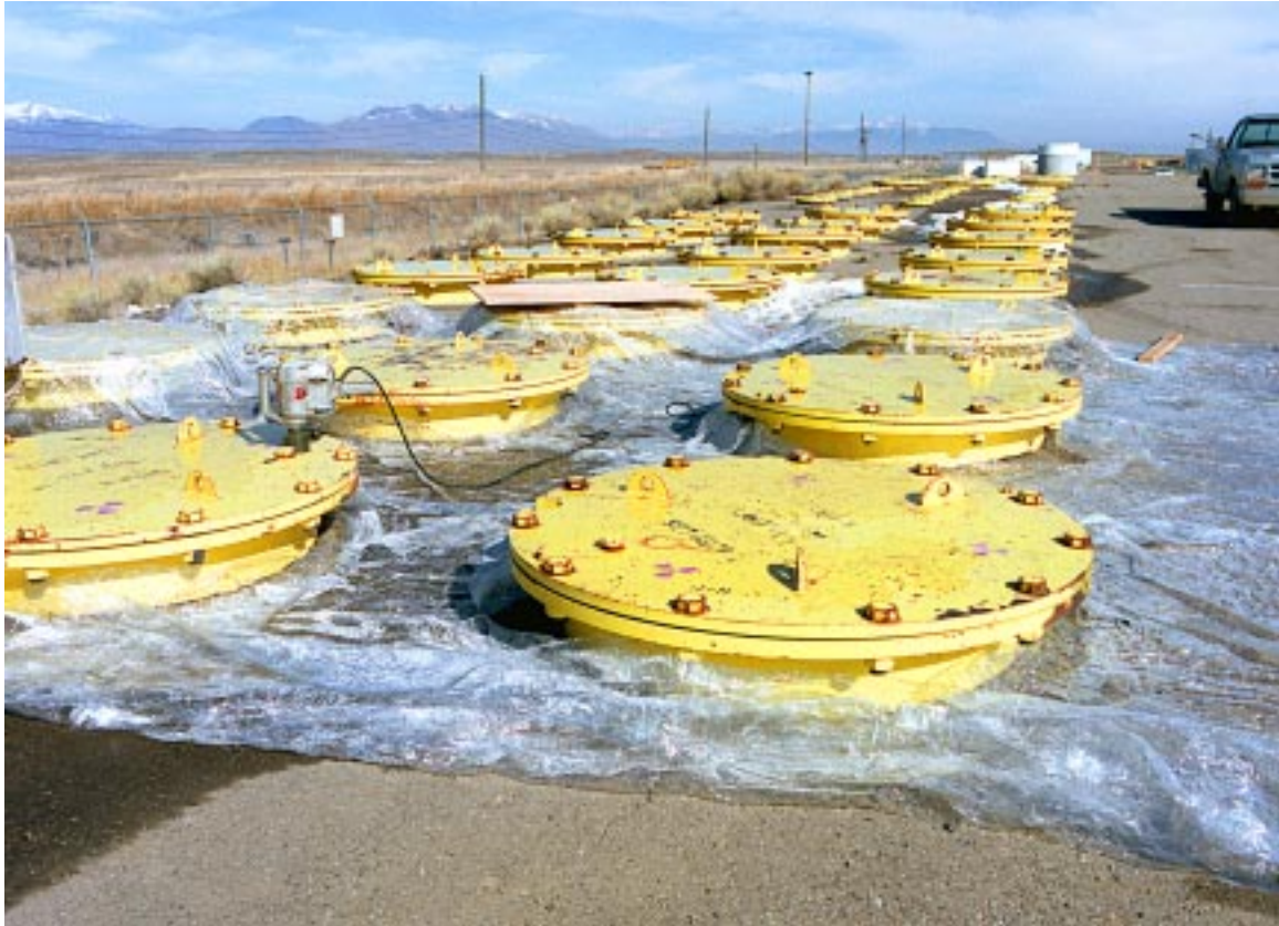
Figure 2. Remote-Handled Transuranic Waste Storage Vaults
