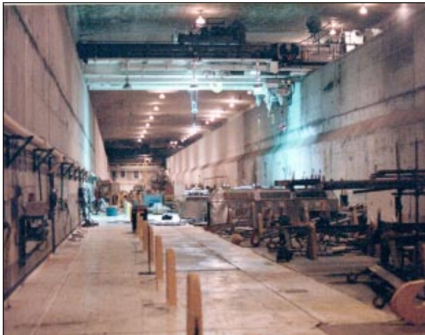
Figure 6. View of the T Plant Canyon, Potential RH-TRU Processing Facility
