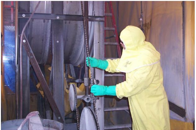
**Figure 4 - Diamond Wire Rope and Pulleys**
