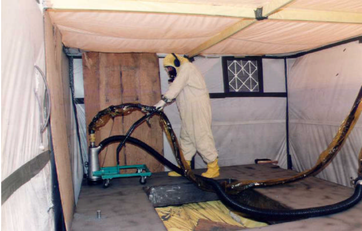
Figure 2. Decontamination of a Shield Door Surface by Abrasive Blasting.
