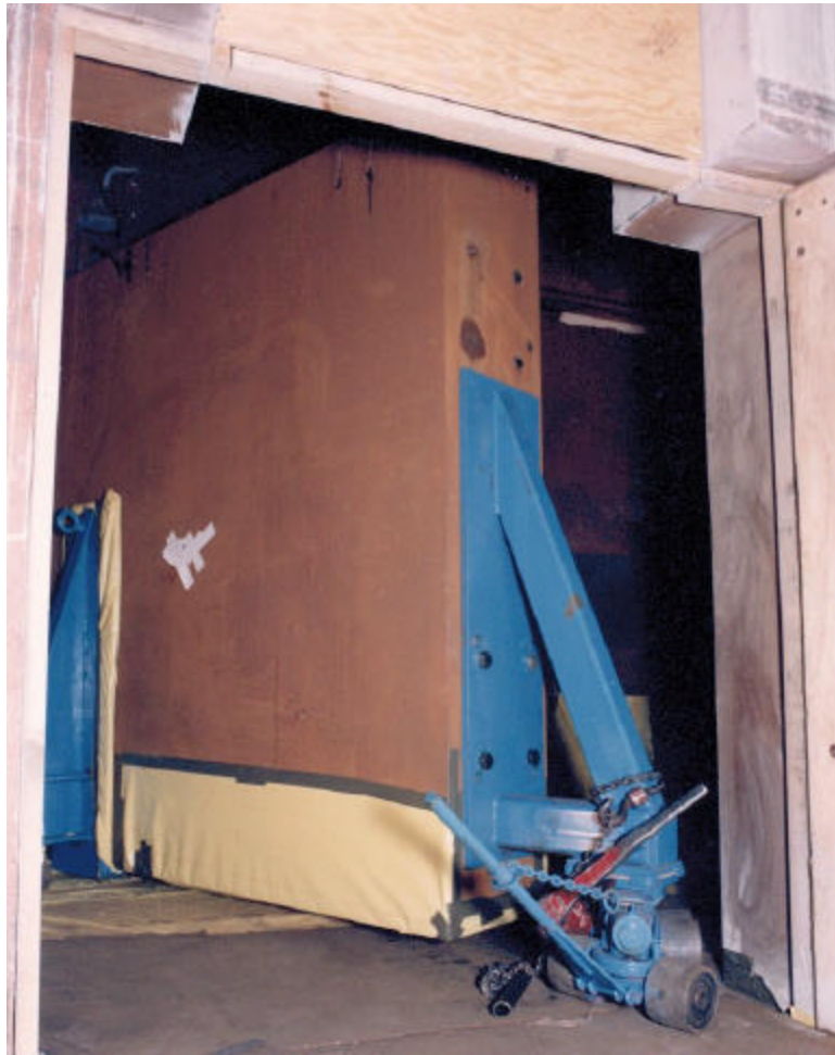
Figure 1. Removal of a Shield Door from the Hot Laboratory Facility.
