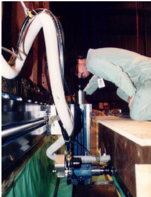
Figure 3. Removal of Contamination Embedded in a Door Edge Using a Portable Mill.
