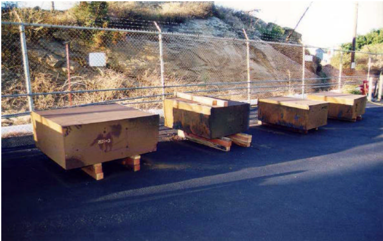
Figure 5. Decontaminated And Size-Reduced Shield Door Sections Released for Recycling.
