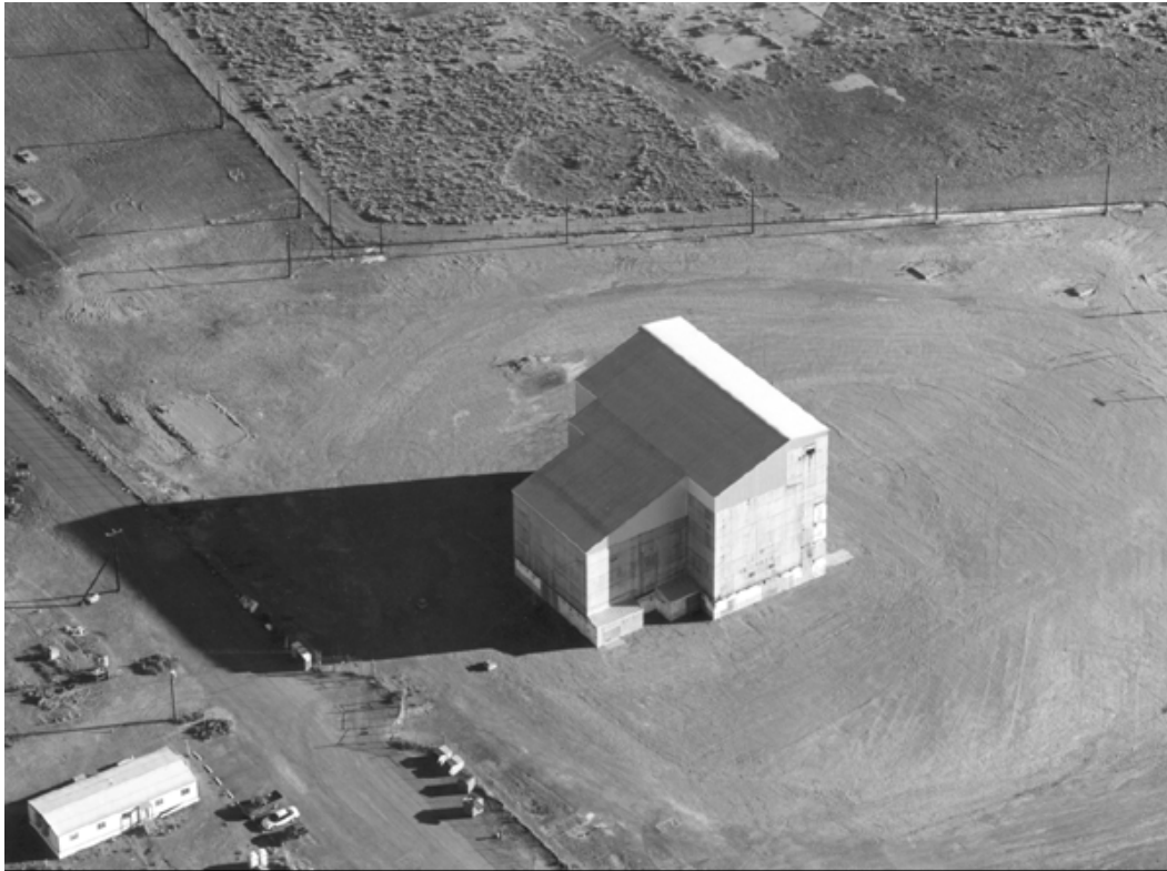
Fig. 3. C Reactor in Interim Safe Storage. (The reactor footprint was reduced by more than 80%.)
