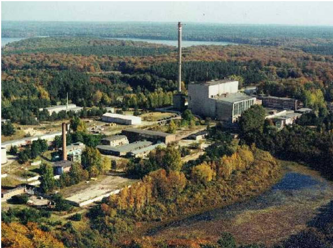
Fig. 1. Nuclear power station Rheinsberg (KKR).
