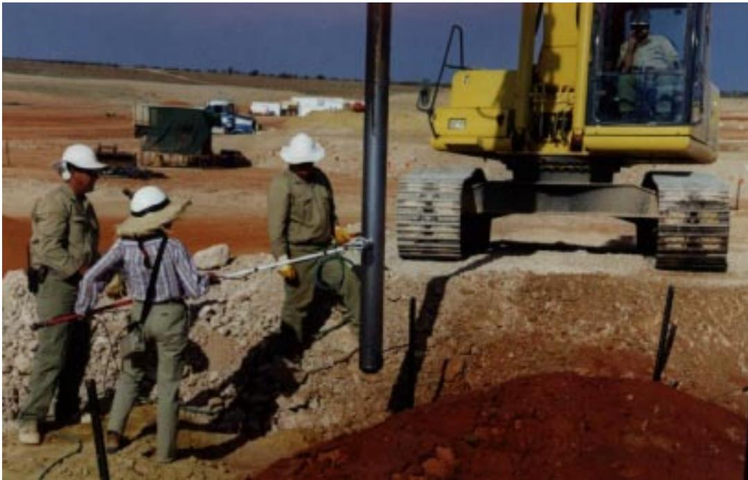
Figure 2. Health Physics check of probe surface during probing of Taranaki Pit 3. Due to the nature of the contamination in the pits and the presence of clean cover soil above the pits, the retracted probe did not normally have significant surface contamination.
