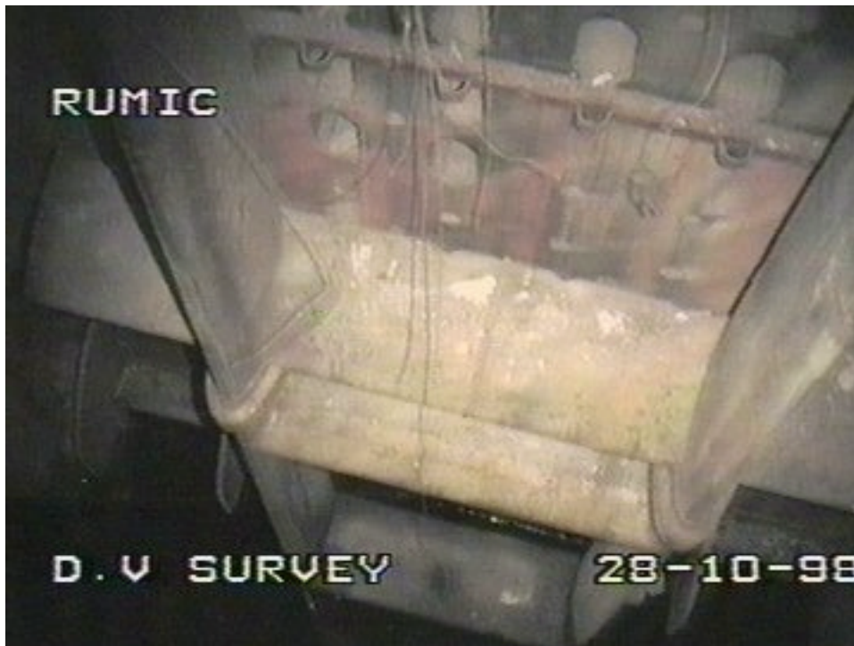
Fig. 3: View of one Burst Slug Scanning Gear.
