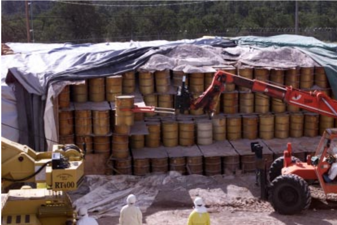
Fig. 1. Retrieval of transuranic waste containers from Pad 4.
