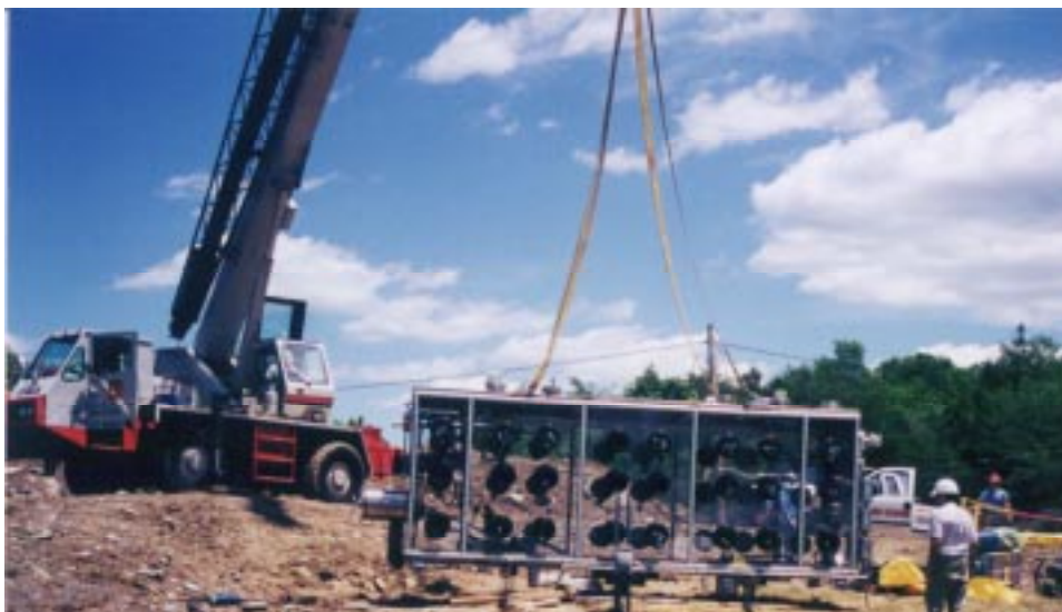
Figure 3. DCM being installed at Tank T-14 Site.
