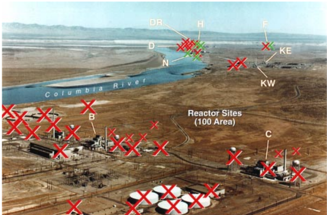
Figure 4. Visible Progress. The “X’s” in this view of Hanford’s reactor areas represent the significant Environmental Restoration progress being made along the Columbia River.
