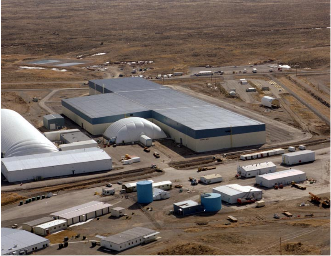
Photo 1. A close-up of the TSA-RE building looking north to south.
