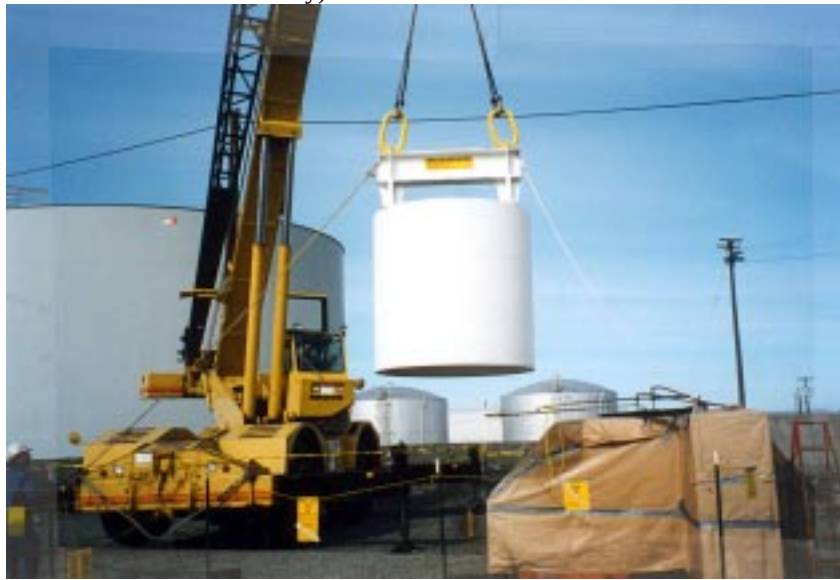
Fig. 4. Removal of HERH Containers.
