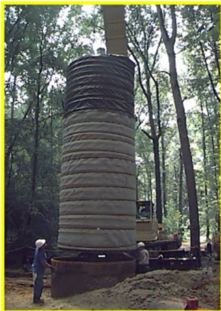
Fig. 3 and 4. The first GeoSiphon well was installed in summer 98.
