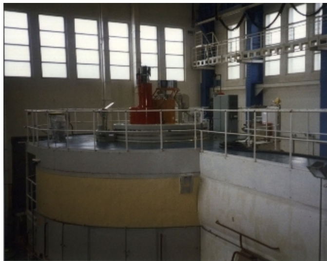
Figure 1. Budapest reactor at the AEKI Institute in Hungary
