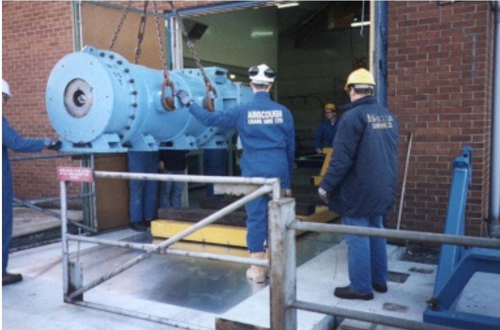
Fig. 4. - Delivery of the Modular Flask to the ICI Site
