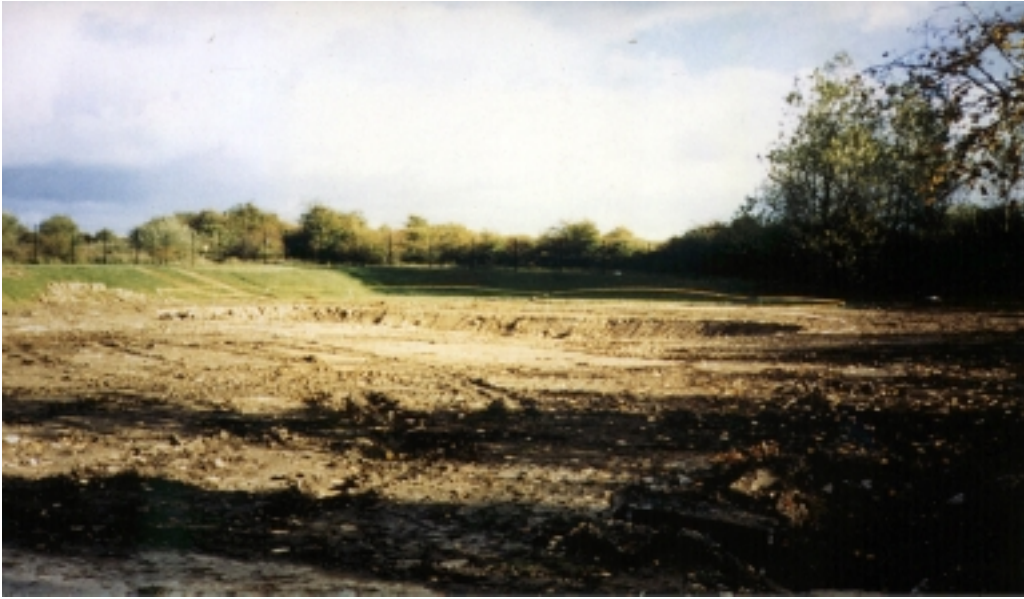
Fig. 2. The URR 'Greenfield' Site Following Delicensing
