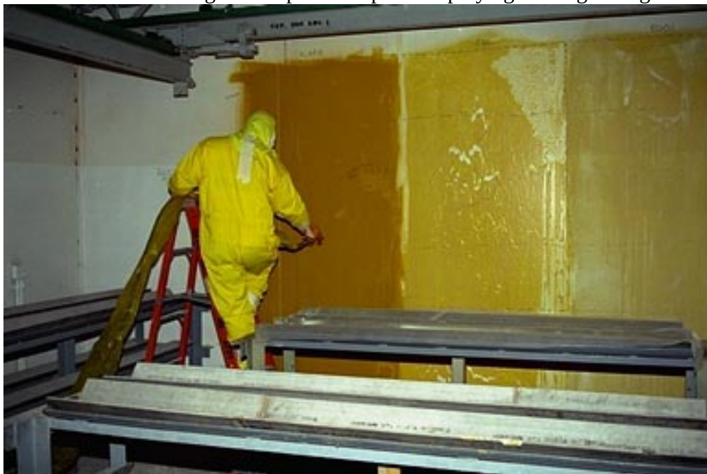
Figure 1. Spray Application of Strippable Coatings
