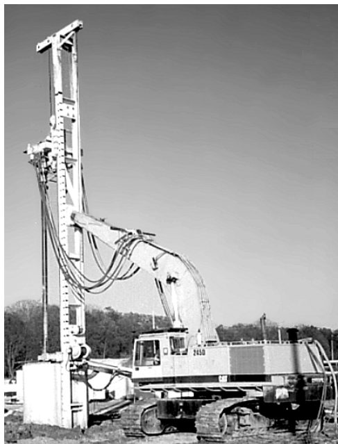
Figure I Soil Mixing Rig
