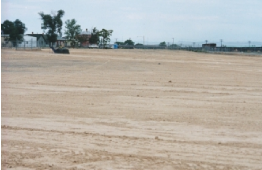
Fig. 4. Site Reconstruction Completed
