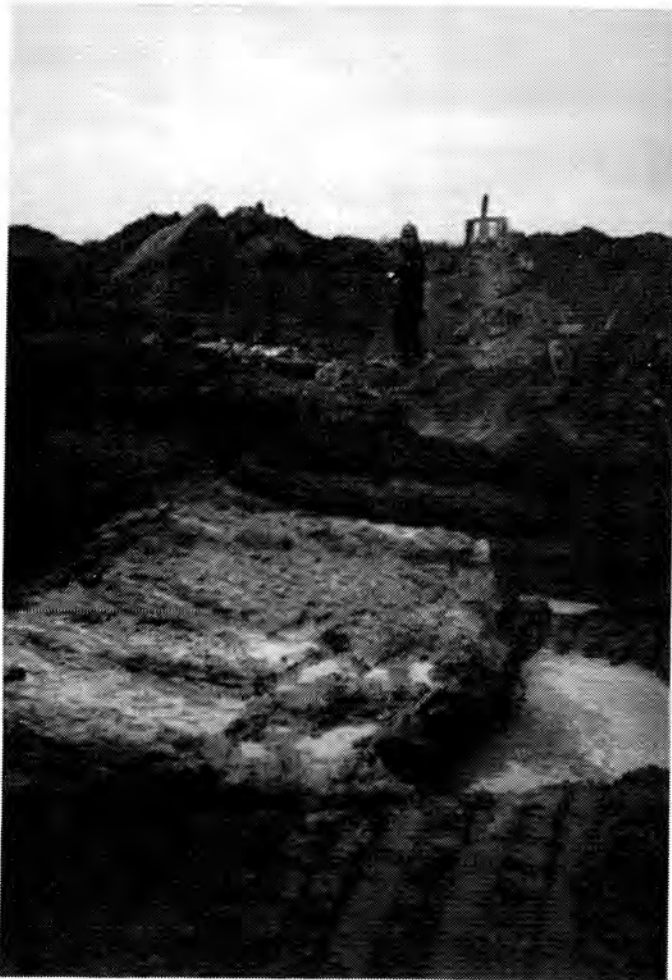
Fig. 4a. Proto type in situ-constructed barrier strip.
