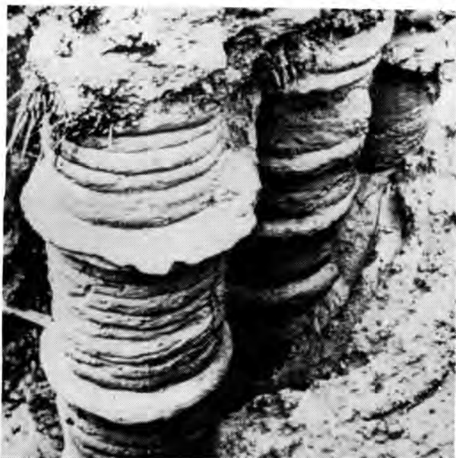
Fig. 1. Example of soil-cement columns formed by jet grouting.
