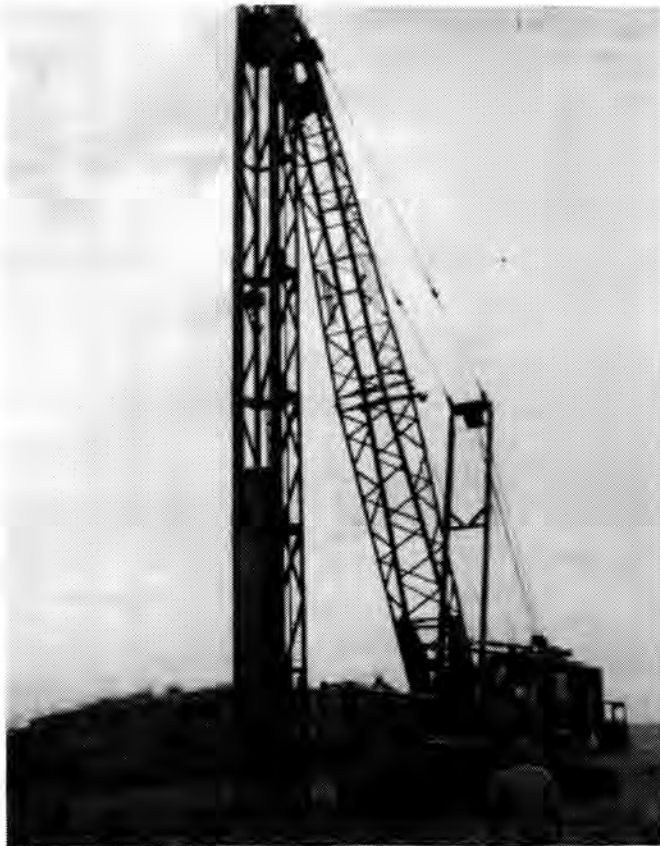
Fig. 6. Diesel single-action pile hammer and leads for primary barrier construction.
