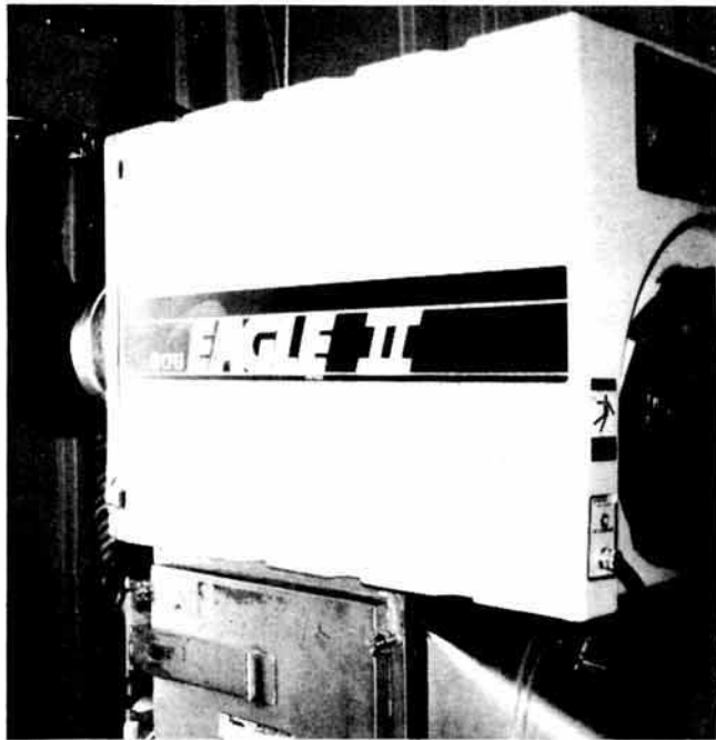
Fig.15. LVRs HEPA Filters.
