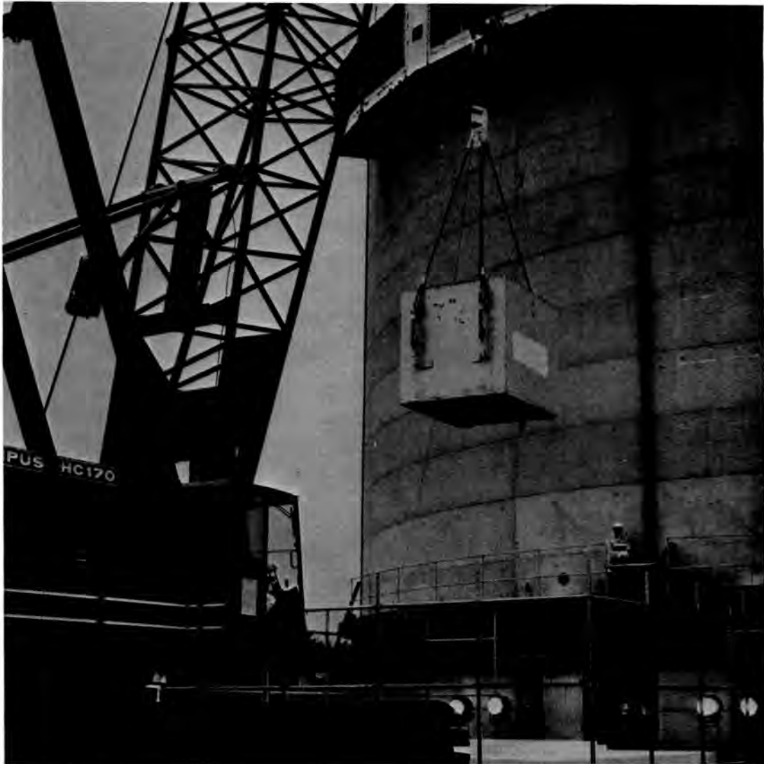
Fig. 2. A 40 te Prototype WAGR Concrete Waste Package Prepared for a Flat Base Drop Test.
