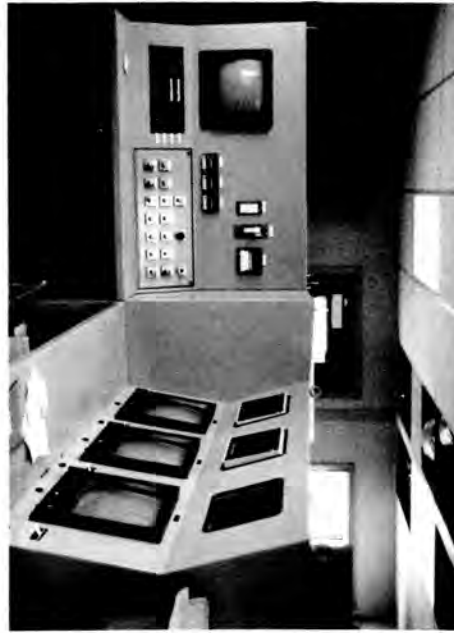
Fig. 7. View of Control Console (LH Section) During Installation.
