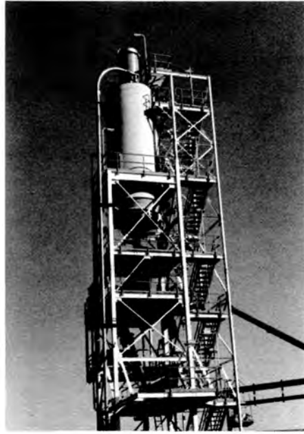
Fig. 3. The Assembled Dry Blend System.
