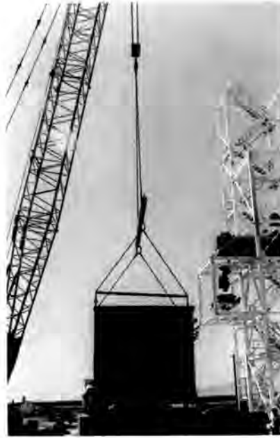
Fig. 5. Setting the LCT/Mixer Module (Right-Partially Assembled Dry Blend System).
