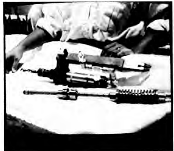
Fig. 4. Guide Tube Cutting Device and Flow Orifice Drill.
