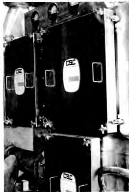
Fig. 6. Access Doors, Bag-In/Bag-Out HEPA and Charcoal Filters
