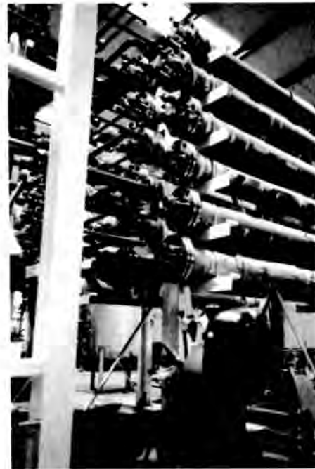
Fig. 6. Connections between Valve Station and HF Modules
