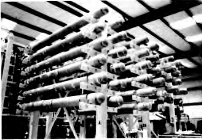
Fig. 5. Rack Mounted HF Modules
