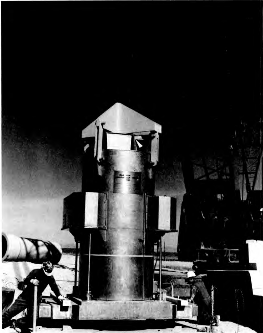
Fig. 6. Soil vault disposal utilizing a 55-ton cask.
