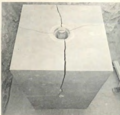
Fig. 7 Post Test Crack Pattern
